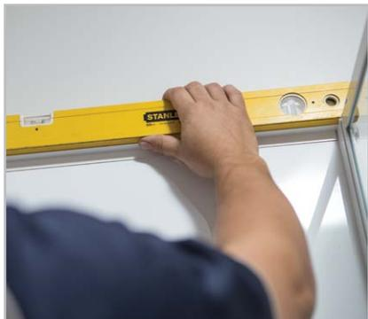
*Attach to the walls (A & B) one at a time ensuring they are level and the slots in the F-Rails are level with the top of the shower frame.*
